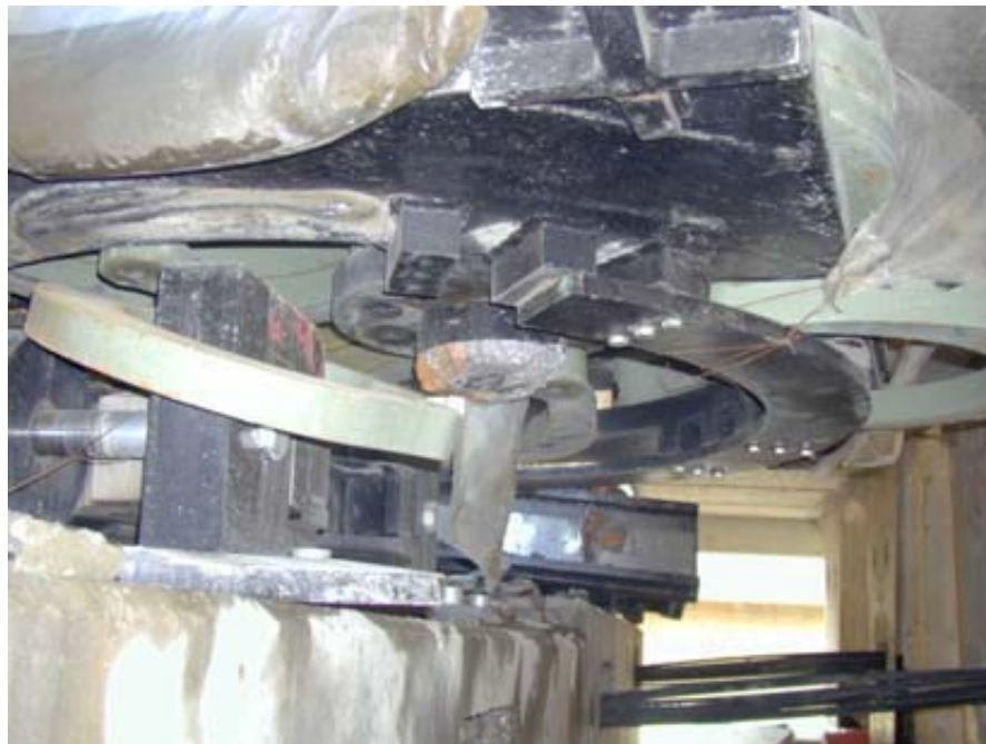
Figure 11. Over-extended "moon shaped" elastic plastic device in the Bolu viaduct [11] due to permanent fault line displacement. These devices were replaced by LRBs
