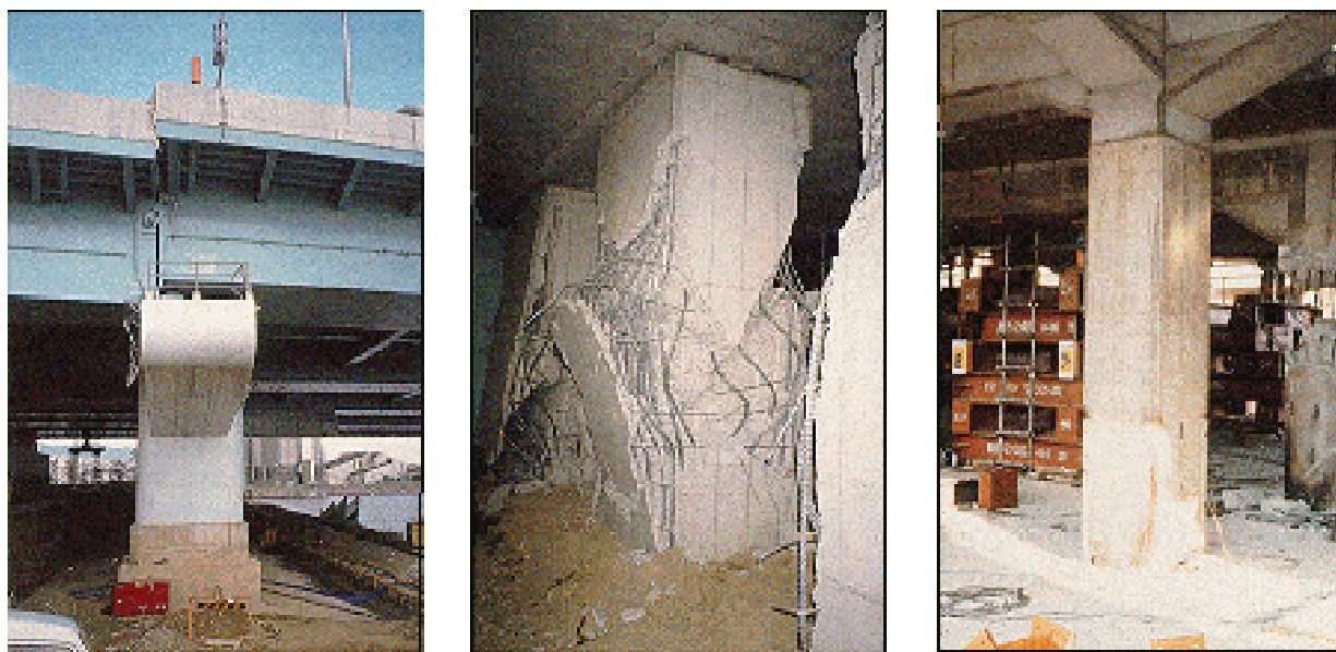
Figure 1. Shear failure of piers of the Hanshin Expressway in Kobe during the Hanshin-Awaji earthquake (from www.fhwa.dot.gov )
