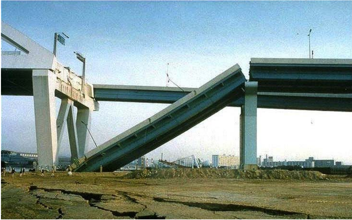
Figure 2. Drop-off of a large steel section of the Hanshin Expressway during the Hanshin-Awaji earthquake (from www.washington.edu )
