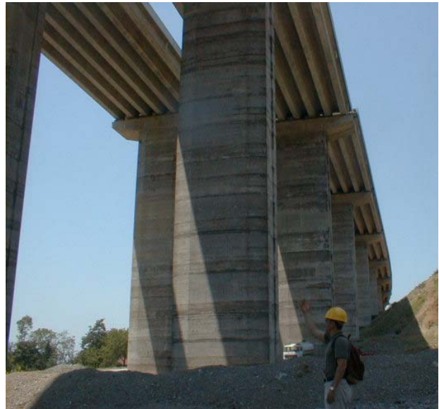
Figure 10. Bolu viaduct with large permanent offset due to fault rupture (from www.purdue.edu )
